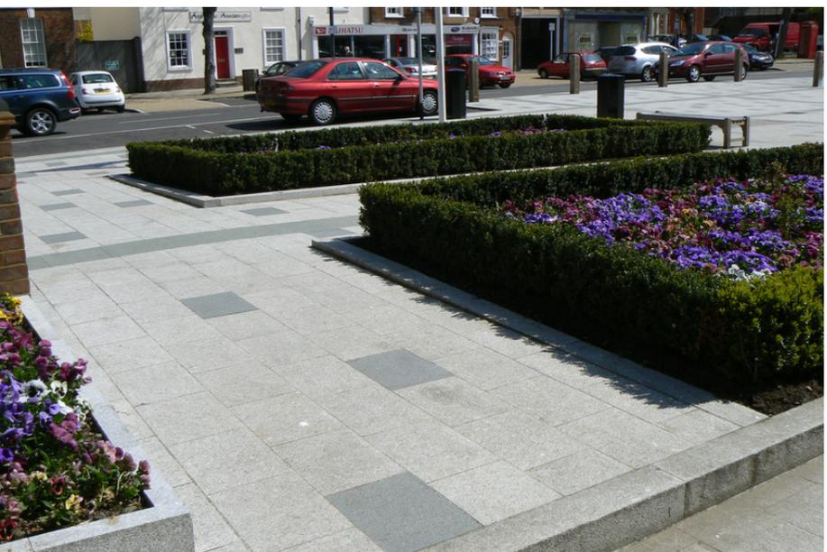
The paved area is around 3000m2 and is set out in a 3 colour mix; silver grey fine picked, mid grey flamed and dark green flamed. We also supplied fluted drainage channels which include 20mm grooves cut on the top surface. All materials were responsibly sourced and supplied within the projects required time-scales.
