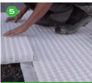
5 installing the ECCOgravel®
