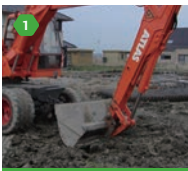
1 perform the excavation works
