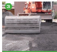
3 compact with vibrating plate
