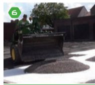
6 placing the gravel
