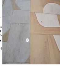
Limestones in general should be assumed to fail under freeze-thaw conditions so should not be used externally unless there is sound evidence of the stone's capabilities. Purbeck stone from a number of the many worked beds has proved -- its worth as paving - quite surprisingly so. Blue Lias, likewise, has successfuly served as paving, but only relatively small quantities of this stone can be supplied.
