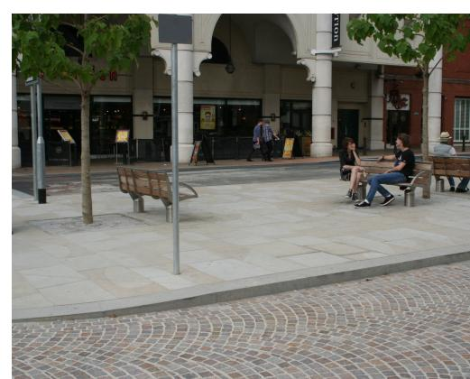
It is visible, but perhaps not immediately obvious, that SuperCEDEC has been used in the tree pits. It is free-draining, yet not readily kicked out over the pavement and it can accommodate growth to the trunk and movement of the roots.
