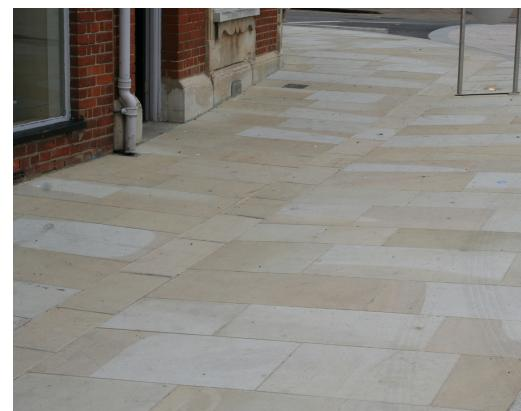
Some details cannot be seen at all such as the 150mm deep Yorkstone flags laid where the beer barrels are delivered but such is the difference that the work has made to the locality that the deliverymen then took special care to unload their barrels on the setts to avoid damaging the flags.
