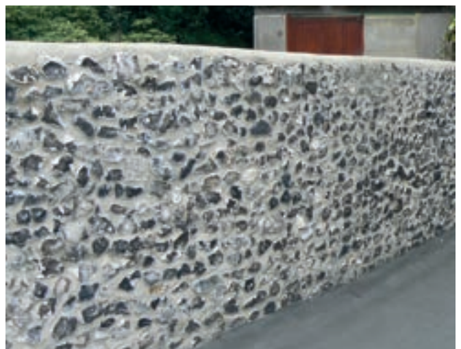
▲ Products: Stone Walling - Knapped Flint
