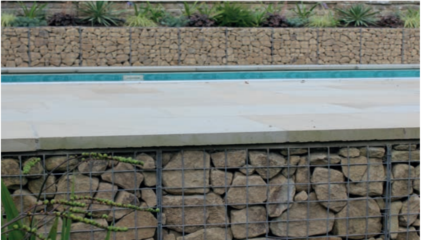
▲ Products: Gabion Fill - Yorkstone
