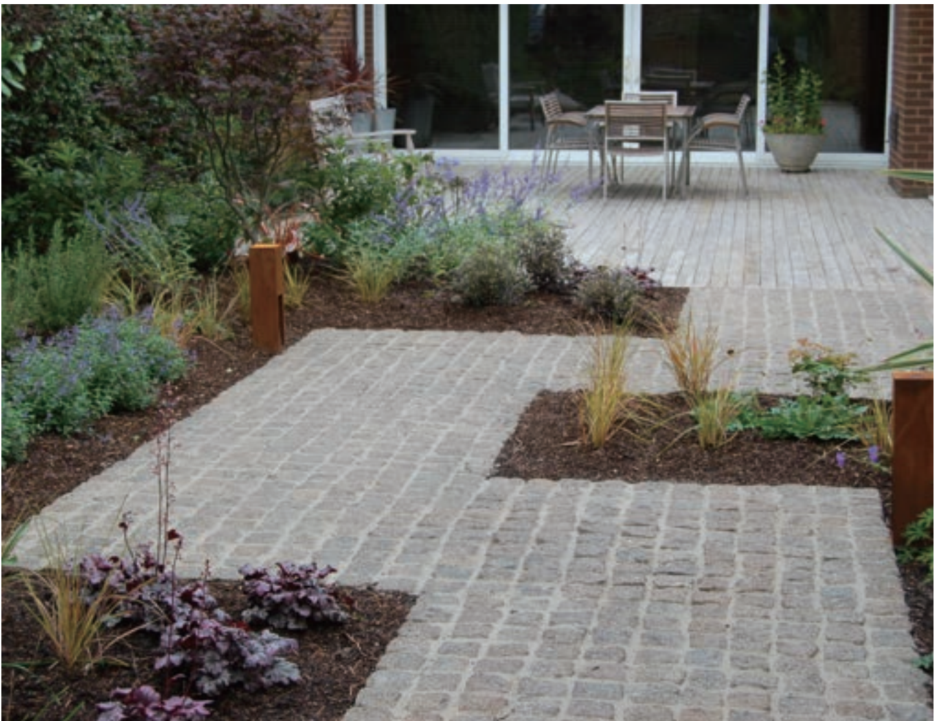
▲ Designer & Contractor: Matt Nichol Garden Design | Creative Gardens & Driveways - Products: Cropped Setts - Yellow Granite
