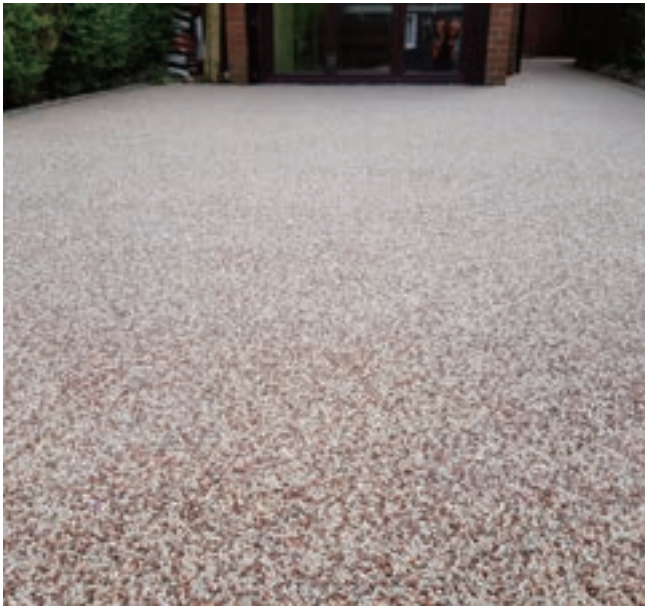
▲ Designer & Contractor: Fern Resin Products: Resin Bound Surfacing - Pearl Blush
