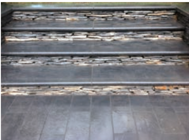
▲ Designer & Contractor: David Greaves Landscape Design & Construction - Products: Imperial Steps & Paving - Black Basalt & Yellow Paddlestone Walling
