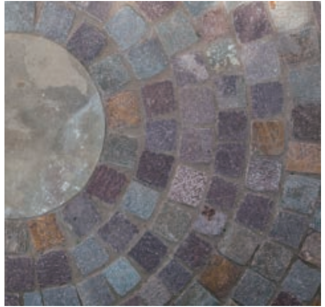
▲ Designer & Contractor: Simon Orchard Garden Design | Hortus Build Ltd - Products: Italian Porphyry Setts *
